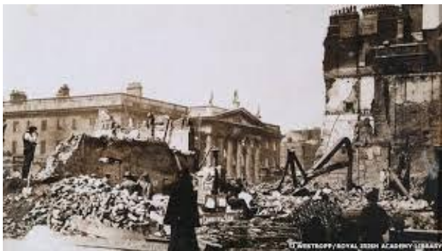
General Post Office in Dublin gutted
