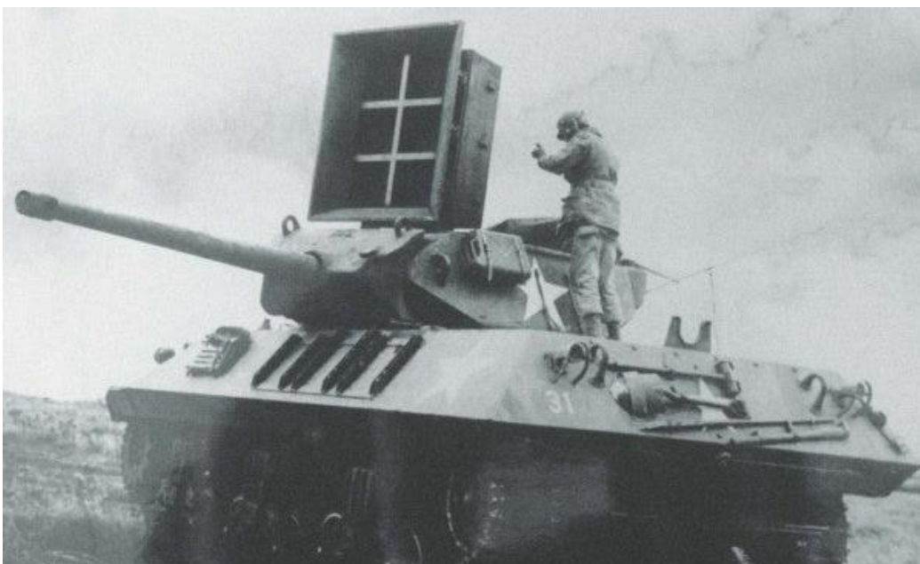
The powerful speakers used to transmit sounds of military equipment and action to deceive the Axis forces
