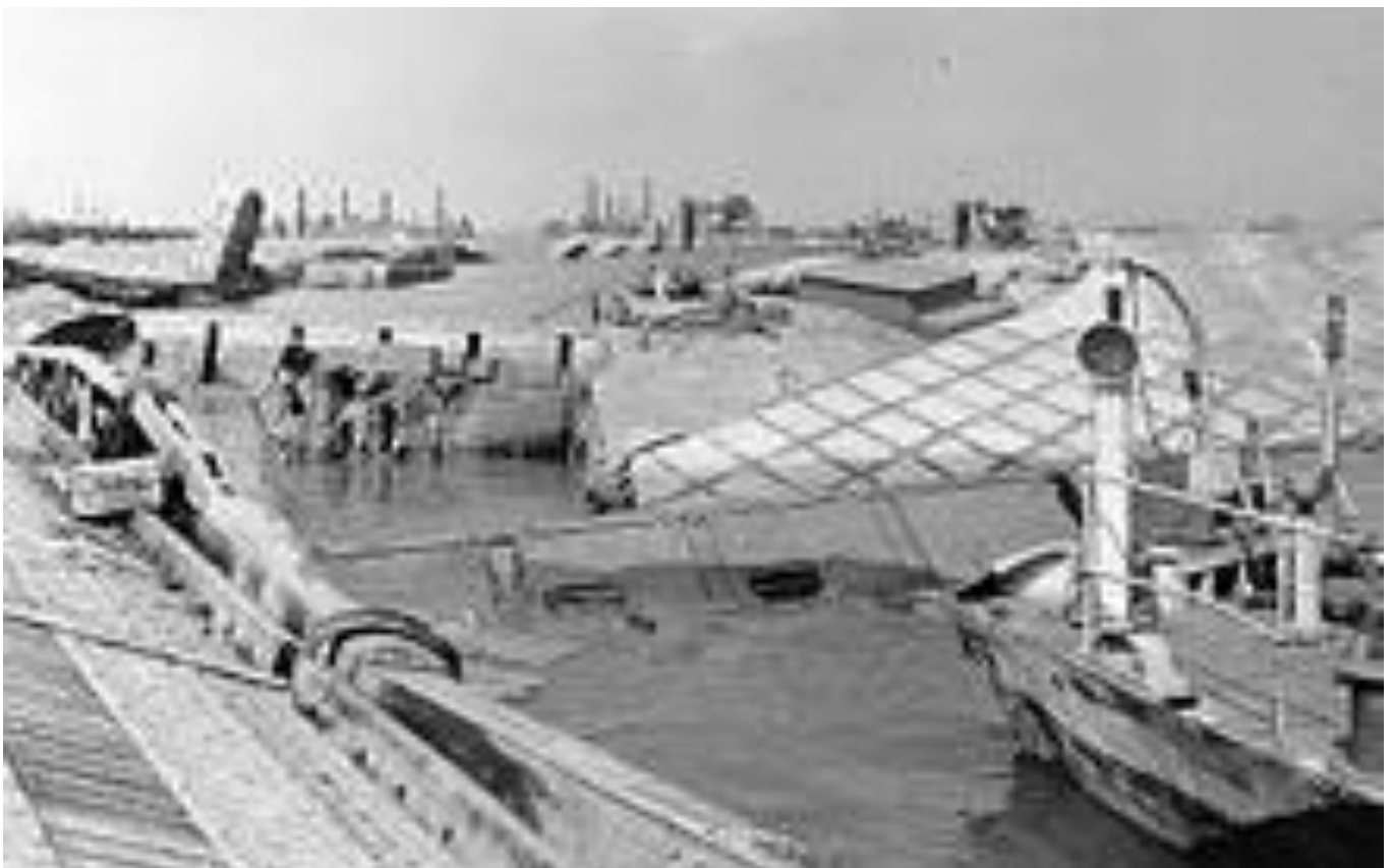
Wrecked pontoon causeway of one of the "Mulberry" artificial harbours, following the storm of 19-22 June 1944
